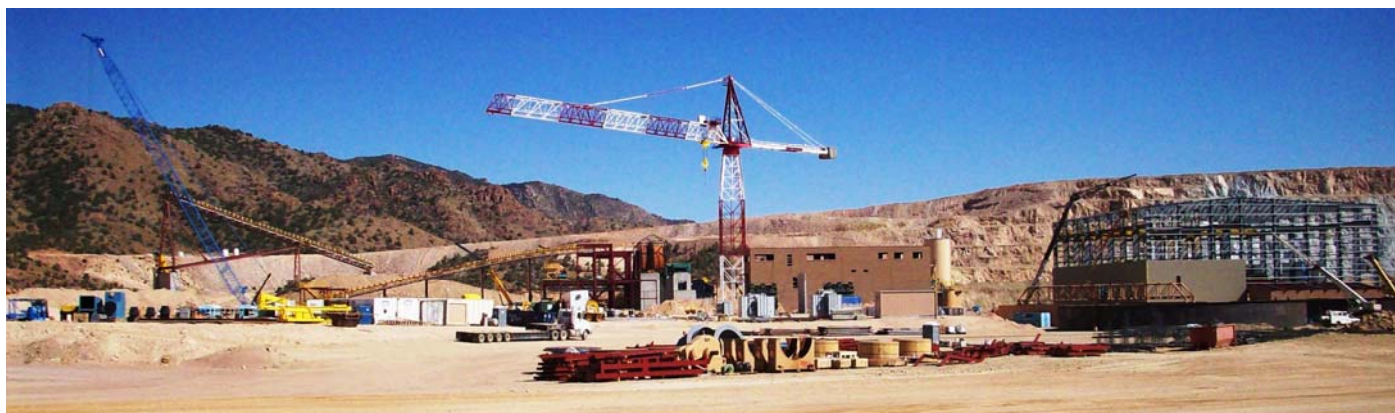
Figure 1 – Mineral Park Project Under Construction, June 2008
