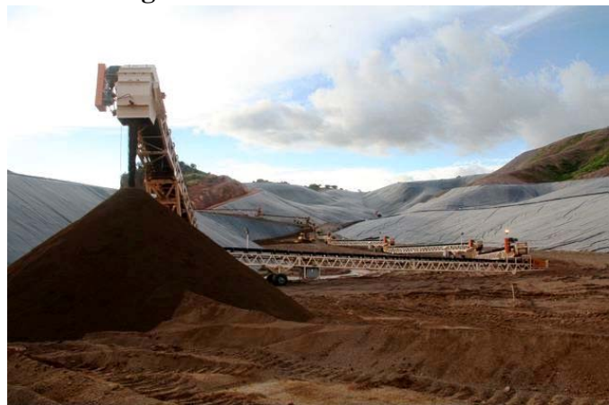
Figure - 4 - Stackers Place Ore on Leach Pad Source: Minefinders
